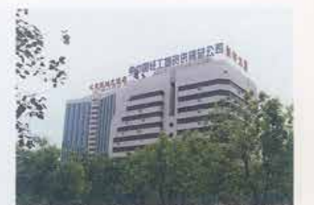
由公司合资建造的亚洲大酒店和新中大厦外景 The outdoor scene of the Asia Hotel and Xinzhong mansion in Beijing built by Century Line with Chinese partner.
