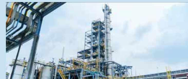
BP 重庆醋酸工厂 YARACO, BP's acetyls plant in Chongqing
